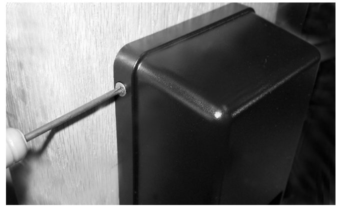
FIG. C: SECURE TOP OF "INSIDE HOUSING"
