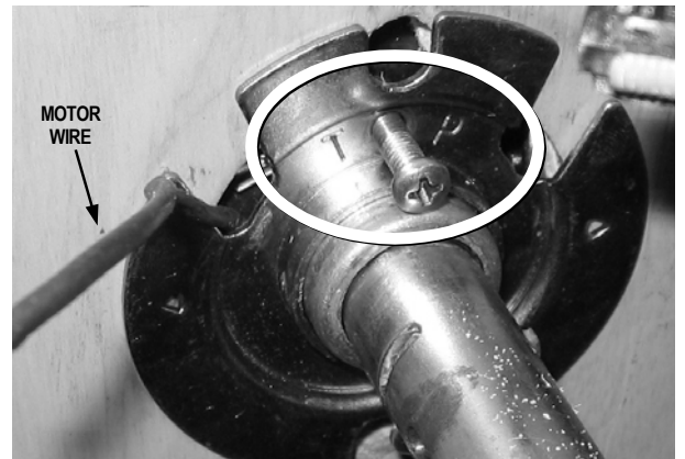
FIG. 12: INSIDE ROSE PLATE INSTALLATION
